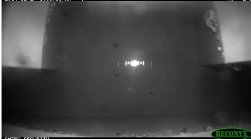
Fig. 9: flooding due to large amounts of water covering the whole bottom of the traps (4).
